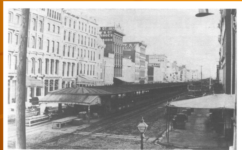
1.3 Market Terminus, Market Street, Philadelphia, 1859 (Courtesy of the Print & Picture Department, Free Library of Philadelphia)
