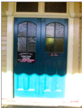
Photograph 12 – Public Bar and Hall for Hire, Lilydale Station
