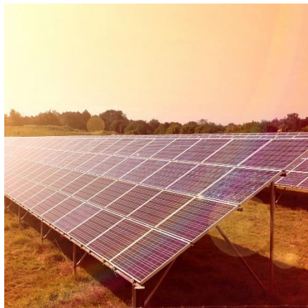
Renewable Energy Innovation Centre - Voices of the Valley
